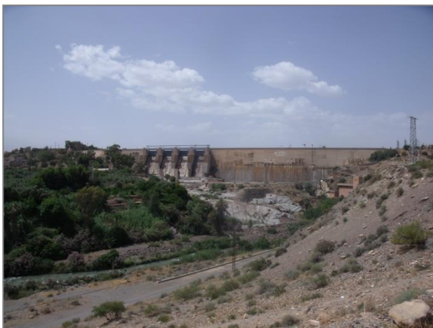
Photo 1 : Barrage Lalla Takerkoust Source: AHT/RESING, 2015
