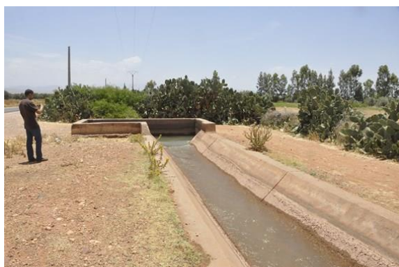
Photo 3 : Le départ de la seguia Sultania Source: Etude Soprolive, RESING, 2014
